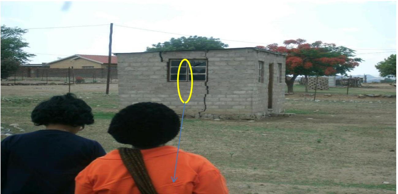
(Cracks on the old Ratanang Crèche building structure)
